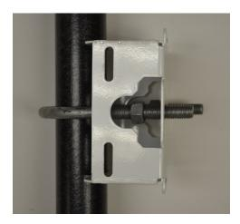
3. Place the angle adapter bracket section on the U-bolt with the open slot connections on the bottom and align it with the pole mount section. Attach with two 1/2 inch nuts. Tighten all nuts to 300 inch pounds (lbf-in).
